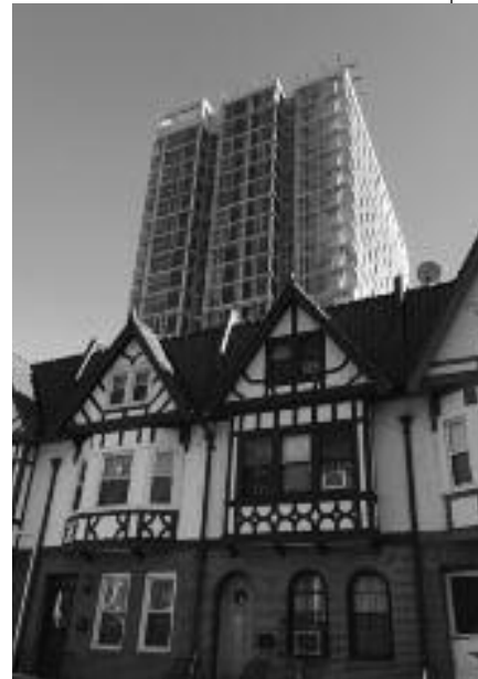
A sun-blocking tall building is no abstraction on historic Chester Court. Many in PLG hope new zoning codes will stop future hi-rises like the 626 Flatbush development.
